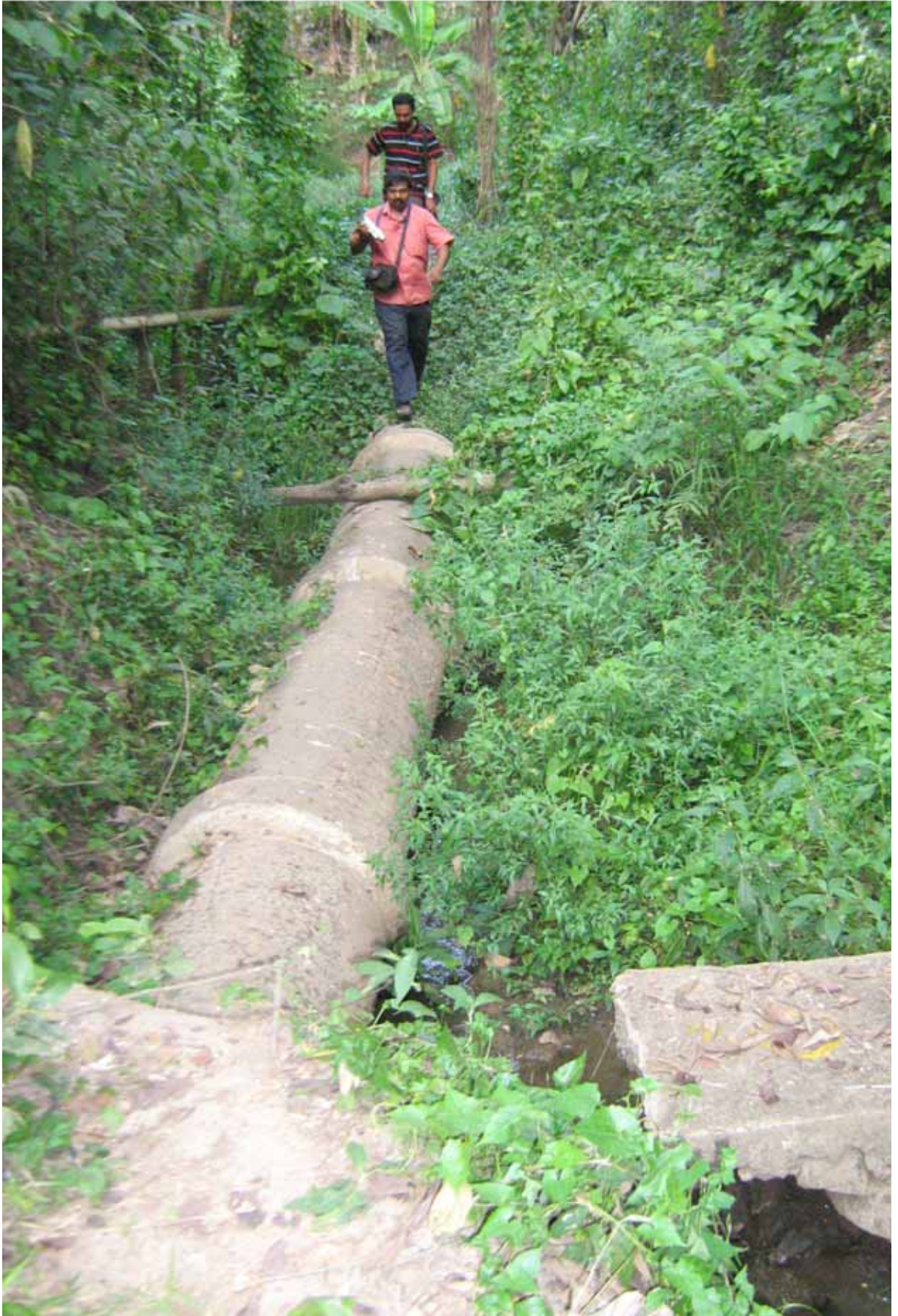
Fig. 11 : Effluents being piped out to Chalakkudy River
